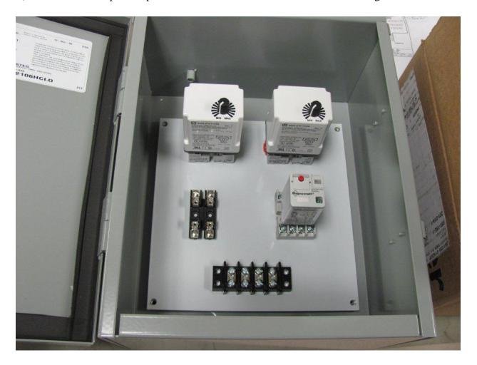
5) With the modification made to the controls, the cooling system was able to be fully utilized as intended in the original design, with a restart that is within about 2 minutes.
