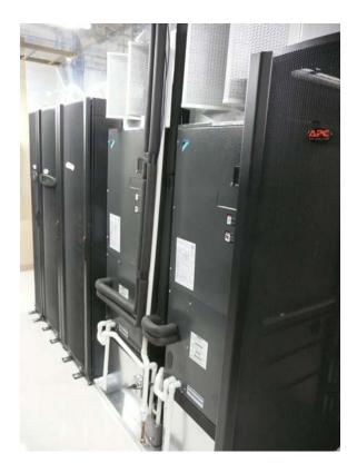
The final design allowed the indoor fan coil units and the outdoor variable flow refrigerant units to provide a high level of cooling for the data center. The energy savings of the variable flow heat pump system is realized, along with redundant system design.
