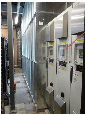
Dedicated Allen Bradley PLCs operate each hybrid dry cooler. Discrete components are used to allow easy field maintenance. Each of the 3 dry coolers are independent in operation. There is a global control to ensure the overall system operates as efficiently as possible.
