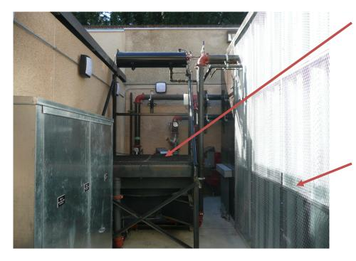
Existing remote generator radiator was not part of this project but had to remain in the equipment yard and required repiping.
