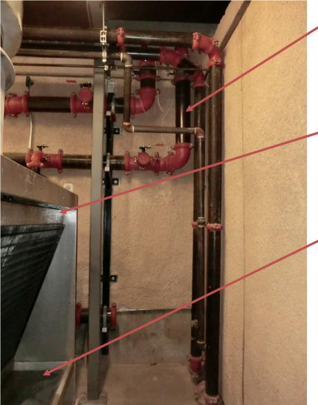
Condenser water piping supporting 100 tons of water cooled A/C units with water side economizers
