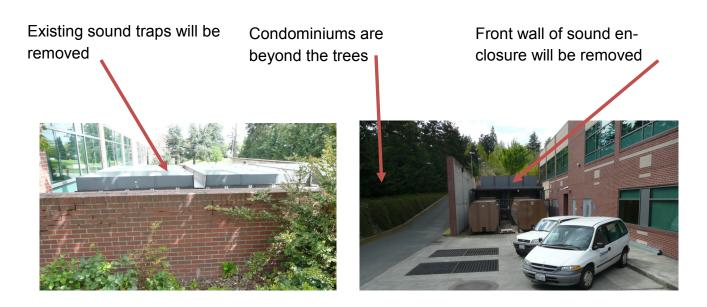
Outside of sound enclosure in mechanical yard. This was replaced by sound baffled air intakes.
