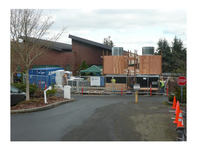
In order for the data center to stay operational for the replacement of the cooling plant, a temporary plant had to be installed. Taking advantage of the modular design of our system, two of the three units were installed for the temporary plant allowing redundancy and the capacity to remove the existing dry cooler plant. The Jaeggi hybrid dry coolers were very compact, and had no vapor plum, this combined with their extremely quite operation made them an ideal choice for the project.
